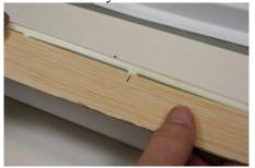
Turn over the paper protecting your work surface so there will be no glue residue to stick to your work. When dry, contact cement will only stick to other dried contact cement, and the bond is permanent so don't let it touch accidentally. Locate a center rib mark to guide your installation.
