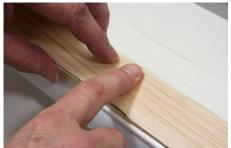
At the center rib, while holding up each end, place the top center edge of the balsa under the top lip (arrow) of the hull. Move to one side, pull and align the top edge of the balsa along the top edge of the hull, pressing as you go.2
