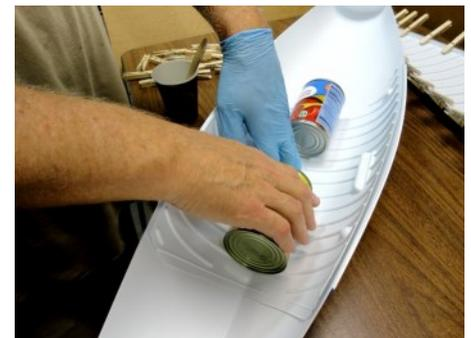
While holding the side together a little, set the Hull Liner into the hull and align it using the two locator bumps and the marked end lines. When you are confident it is in the proper place, set two 15 ounce cans of vegetables into the Hull Liner as shown.
