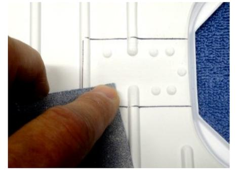
After the Mast Step Backer is glued in place, the Upper King Post Mount is glued over it on the underside of the deck. Set the mount in place and mark its outline on the underside of the Deck. Now sand this area. OK to sand the bumps.
