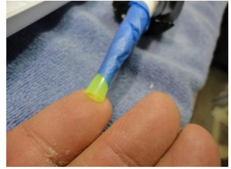
Lightly round just the sharp edge of the spout at the end of the caulking tube. Push the slit-end of the straw onto the caulking tube just past the end of the slits. Carefully tape to leave no gaps for the sealant to ooze out. Pinch the end of the straw to make it flat so it can slide into the Deck groove. If it comes out of the groove while you are applying sealant, take a paper towel and pinch it again to help it go back into the groove.
