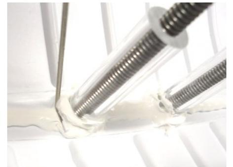
Remove the Crossmember, Keel Tubes & Keel Shoe. Install the two keel tubes. Put a bead of sealant along the center of the hull at the Keel Shoe outline. Just a 3/16" bead but put more around the grooves of each of the tubes. Use a bent wire to work the sealant into the grooves filling them. **Important** to get the sealant completely around the grooved part of the two acrylic tubes. This will form a seal between the tubes, the shoe and the hull so the Keel Mount will not leak.
