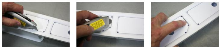
Score along an opening, lightly the first time and with a little more pressure the 2nd or 3rd time. If you knife falls through the slit, tilt it sideways to pull it free. Press on one end flexing the plastic until it separates.
