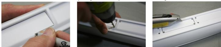
Make the bottom mark about 1/16" ABOVE the pencil line. Drill the four corners of each opening with a 3/16 inch drill. Score the four sides of an opening. It is thicker at the bottom line. Additional scores there. 5
