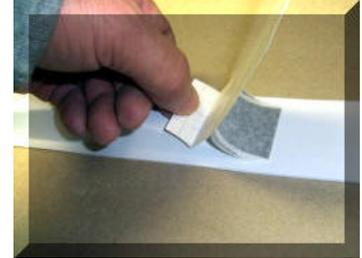
When it is aligned, press across the front and begin to peel the backing paper off.
